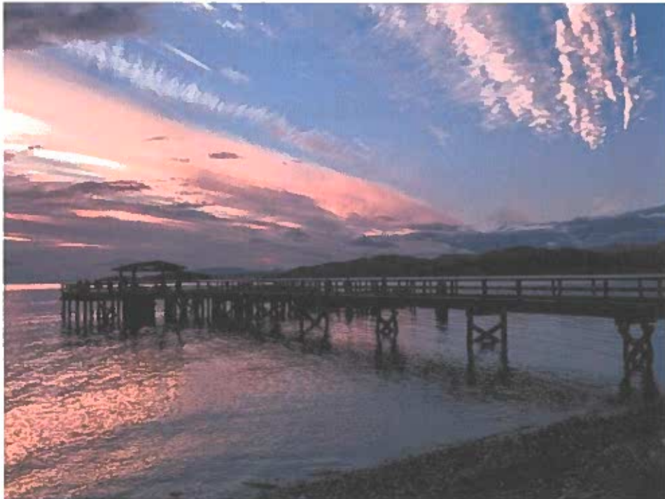
Davis Bay Pier
